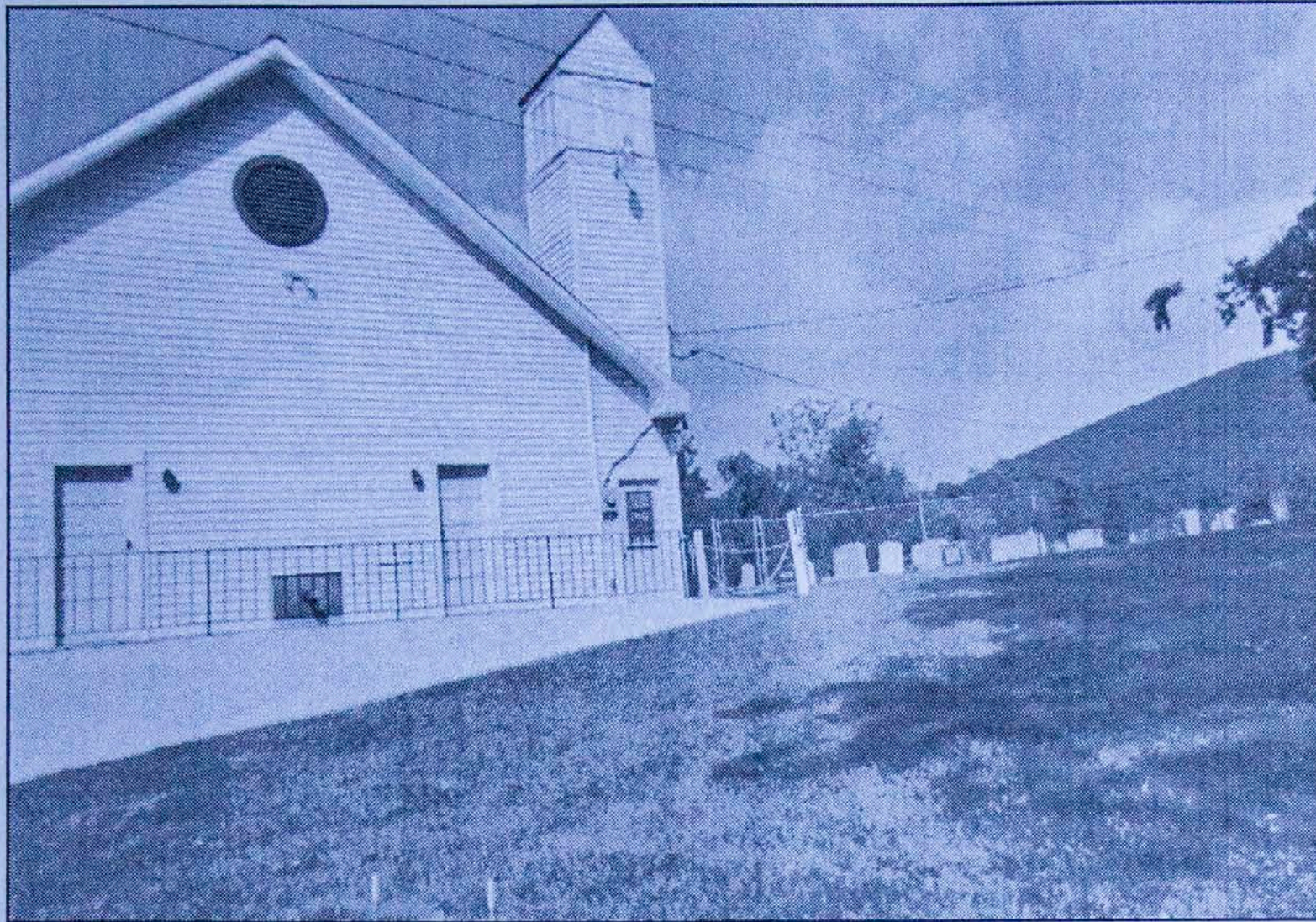
The top photo of the Shockeysville Church shows the bell tower after it was repaired and remodeled in the Summer of 2004.
